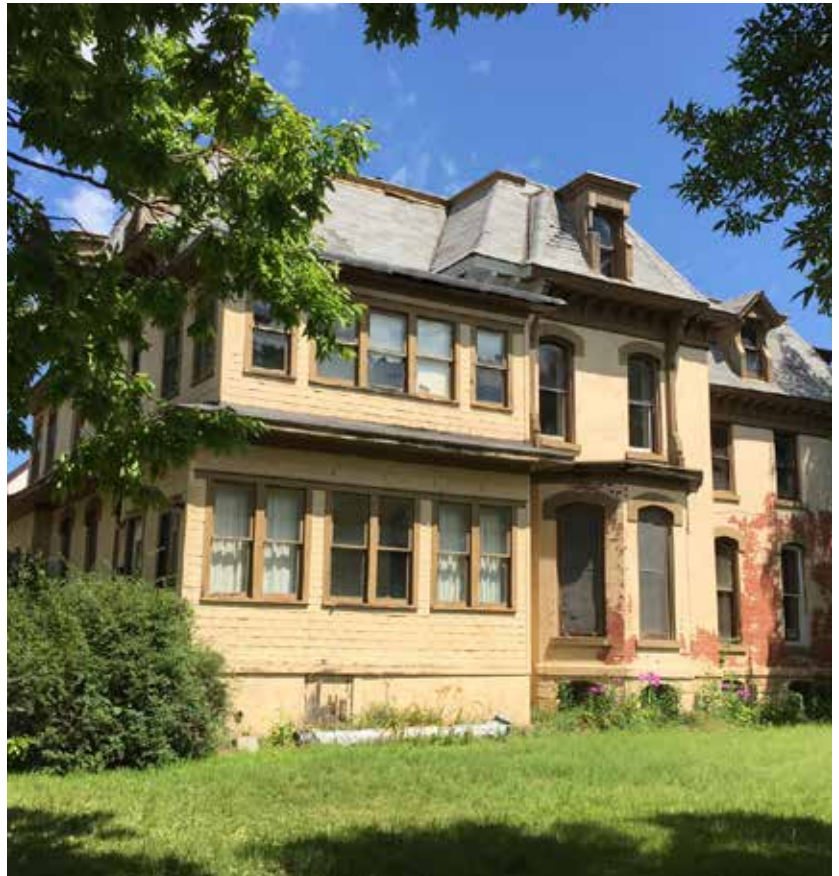
La Crosse residents long used to seeing this version of the Cargill-Pettibone house have cheered on the restoration, especially as a gabled roof and detailed porches were rebuilt.
