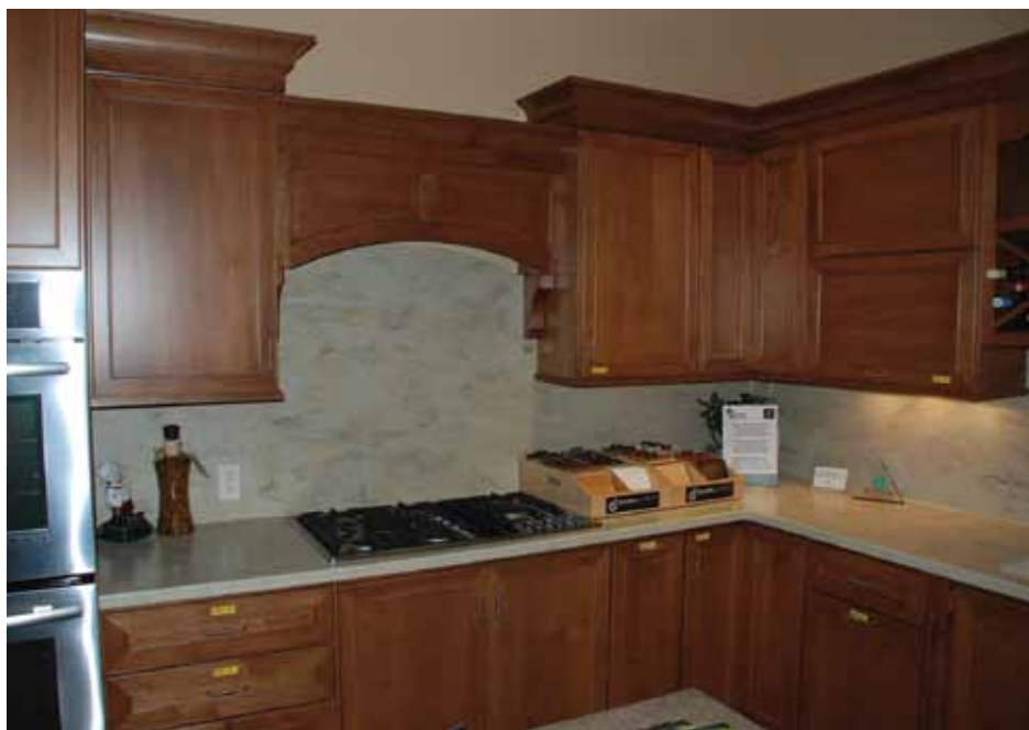
Corian countertops with a full-height covered backsplash are a practical yet attractive option for a kitchen makeover.
